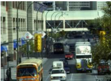
Picture 2 - This Plus 15 bridge in Calgary actually has three stories and is completely glassed in.
